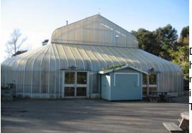
During the past 15 years the opacity of the polycarbonate has increased and therefore light transmission has been much reduced. Energy is now provided from the recently installed solar panels that can be viewed at the rear of the Tropical House.
